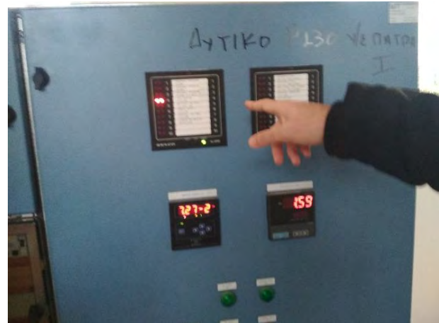
Figure 8-6: Submarine cable monitoring equipment at Rio site
