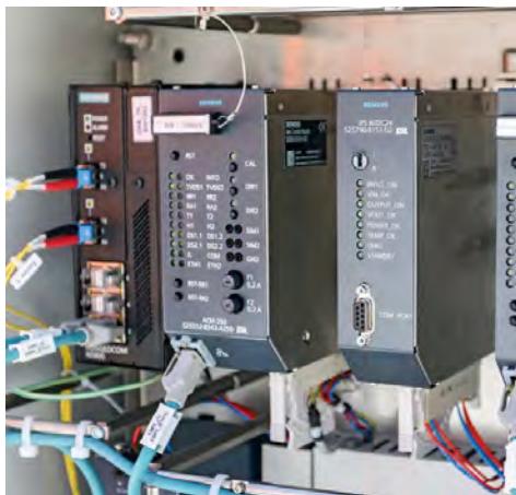
Figure 3-29 EULYNX Object Controller
