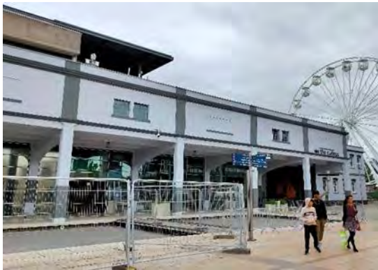
Figure 4-11 WTC balcony area
