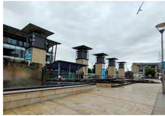
Figure 4-12 MSq Towers 4, 5 and 6
