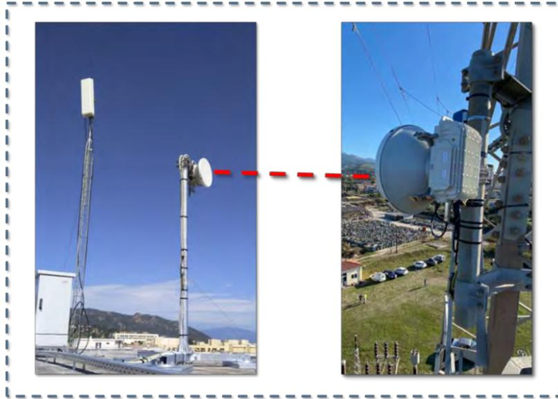
**Figure 4-41 Pictures from the backhaul equipment installed at UoP premises and ADMIE poles for the transport network interconnecting ADMIE facility (the red dotted line indicates LoS)**
